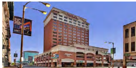
Hampton Inn Gateway Arch 333 Washington Ave., St. Louis, MO (314) 621-7900
